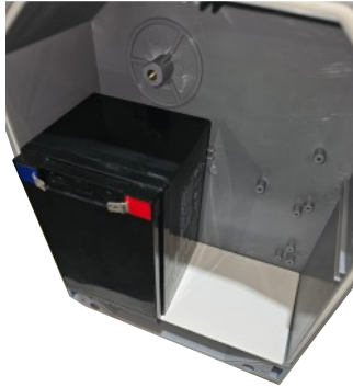
First battery placed in position
